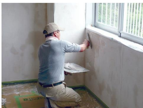
**Fig. 12 Application of interior finishing material that contains HASClay**
