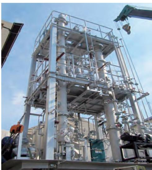
**Fig. 17 Bench plant of CF-HIDiC under installation<sup>[10]</sup>**
