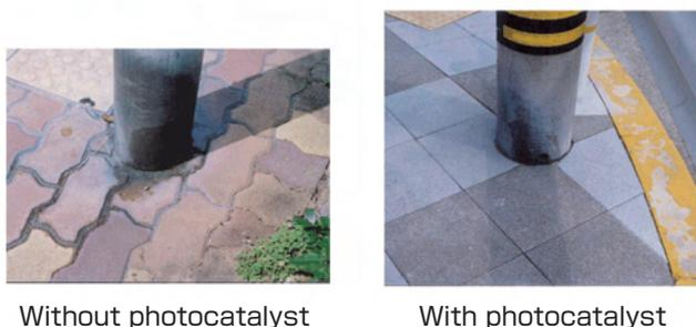
Photo 3. Antifouling effect on surface of photocatalytic permeable block (right).
