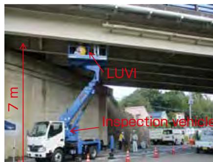
Fig. 12 Scene of fatigue crack inspection in the welded part of a steel bridge
