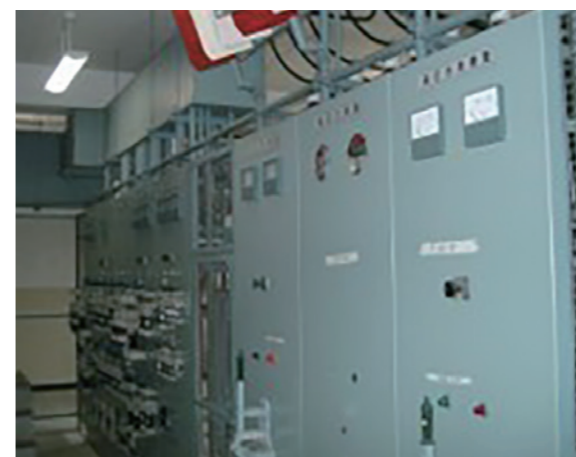
Before substation facility renovation
