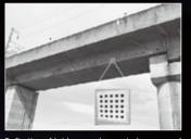
Deflection of bridges can be precisely measured by analyzing digital images. We also develop novel diagnosis technology that can reduce time and labor by integrating information technology such as AI and robots into inspection.
