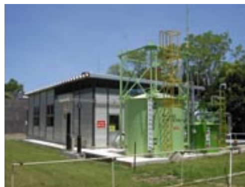
An outer view of the semi-pilot plant
