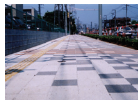
Photo 2. Photocatalytic materials spread out on a street
