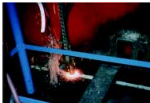
Seawater flushes into the float during cutting operation.
