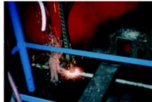
Seawater flushes into the float during cutting operation.
