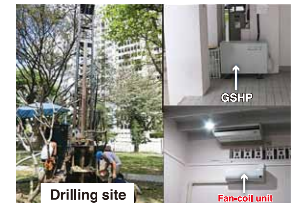
Ground-source heat pump (GSHP) system installed at Chulalongkorn University, Thailand
