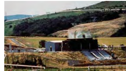
Geothermal power plant repowering with biomass
