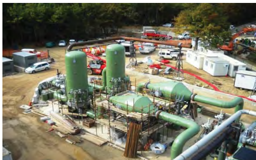
Steam separation system
