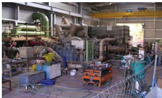
Main machinery erection
