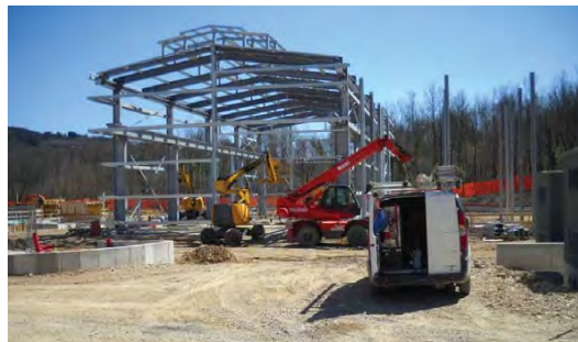
Building machinery erection
