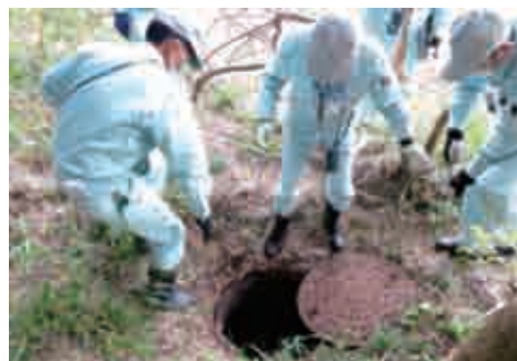
Drill for checking the flow route into the public water system
