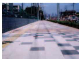
Photo 2. Photocatalytic materials spread out on a street
