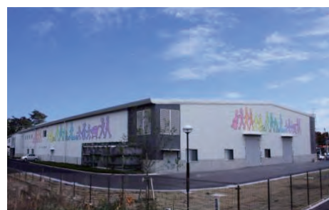
Exterior view of the Robot Safety Center
