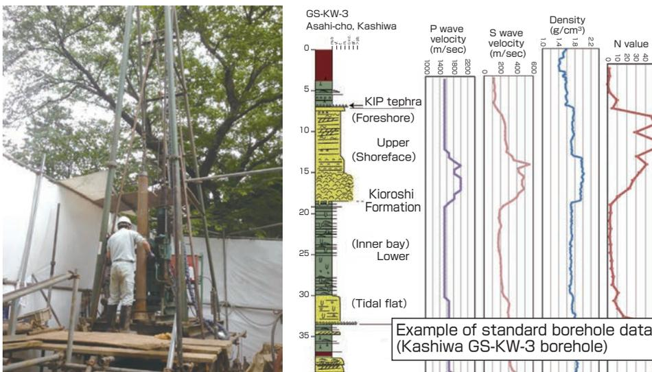
**Fig. 4 Drilling survey and standard borehole data**
