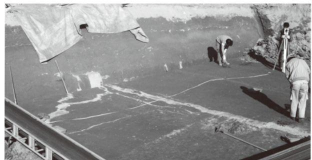
Fig. 2 Traces of liquefaction at the Kizugawa Riverbed Site.
