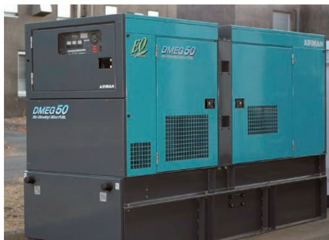
Photo 2 Bio-brened DME generation system
