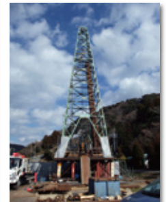
Drilling exploration of a hot spring system in the Minami-Izu area
