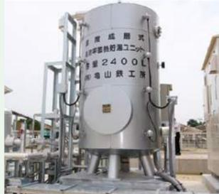
Temperature stratified hot water storage by Kameyama Iron Factory Inc.
