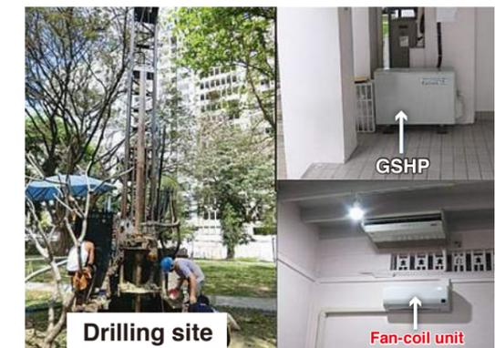
Ground-source heat pump (GSHP) system installed at Chulalongkorn University, Thailand. Facility at Chulalongkorn University in Thailand used to demonstrate the possibility of cooling operation through the GSHP system in Bangkok. \*GSHP: Ground-Source Heat Pump
