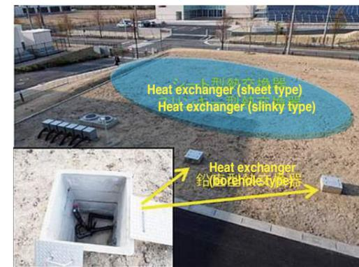
FREA Ground-Source Heat Pump System Demonstration Area. This GSHP system uses a sheet-type heat exchanger and a Slinky-type heat exchanger installed at a depth of 1-2 m and a vertical-type (borehole type) heat exchanger installed at a depth of about 40 m.
