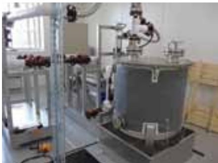
Examination device of hot spring system
