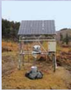
Status of installing the three-component seismometers
