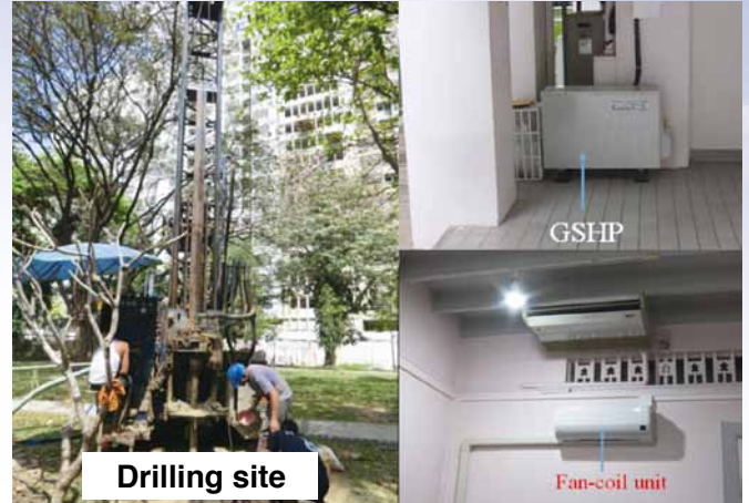
A ground source heat pump (GSHP) system installed at the Chulalongkorn University, Thailand A facility at the Chulalongkorn University in Thailand was used to demonstrate the possibility of cooling operation through the GSHP system in Bangkok. *GSHP: Ground Source Heat Pump
