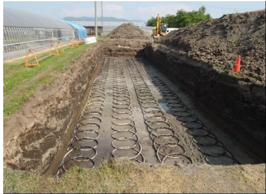
Installation of Horizontal GHE
