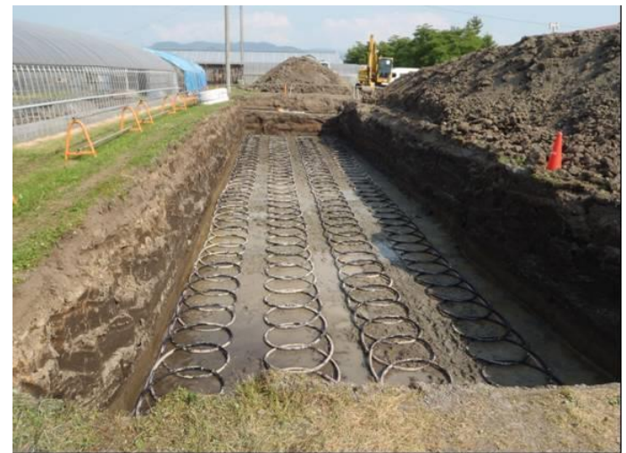
Installation of Slinky-coils (Aomori, Japan)
