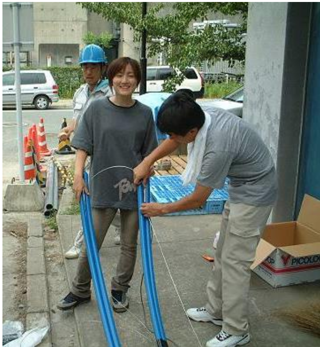
U-tube with Optical Fiber Sensors
