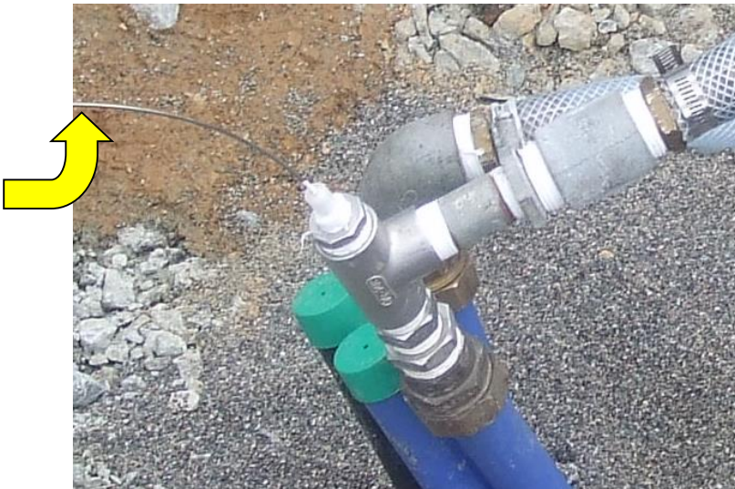
Optical Fiber Sensors in U-tubes
